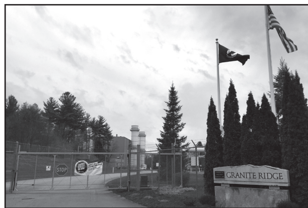
Workers at Granite Ridge Energy first voted to join IBEW Local #1837 in a National Labor Relations Board election in 2006.
